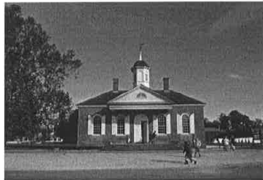
Historic Williamsburg Courthouse
